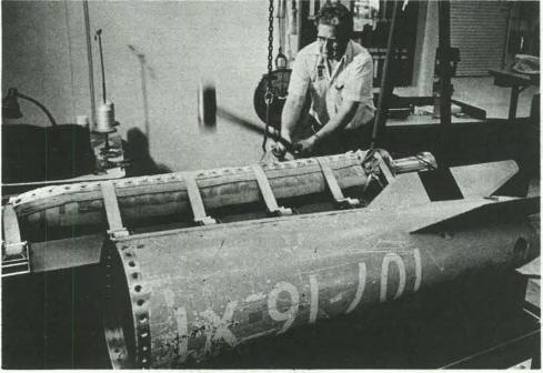
PACKING yards and yards of material and fittings so that it fits into small, confined space (foreground) sometimes takes not-so-gentle touch. Oley Olson variously employs a lace-and-tighten technique and a multi-ton hydraulic press to this end. Sledgehammer and, occasionally, a baseball bat are used as well to bring packed chute to firmness of solid oak.
